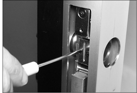
Fig. 4c: Secure interface cylinder to lock
