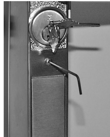
Fig. 5c: Turn key counterclockwise and tighten the cover screw.
